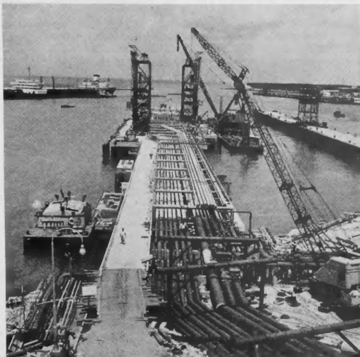
STRUCTURES FOR free-standing loading arms and the arms themselves have been erected on Lago's No. 3 Finger Pier. The new pier virtually looks as it will when fully completed. Most piping, left, has been installed out to the free-standing loading arms on the two structures, center, have been undergoing tests. The project sparked remote-control gates, right, at gate No. 2. The guards will also operate gates to the pier access road.
